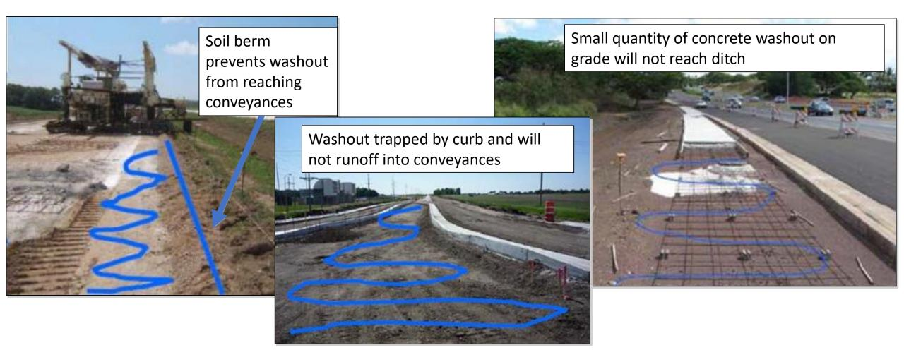
Washout occurring on grade shall not runoff into surface water or stormwater conveyances (inlets, curb flow lines or ditches)
